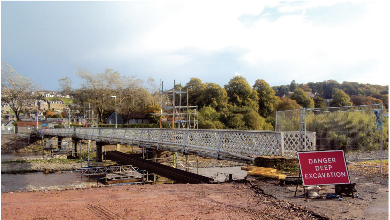
Selkirk Flood Protection Scheme – Temporary bridge works
