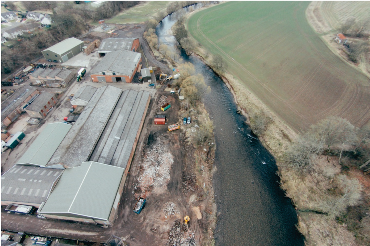
Brechin FPS – Construction works
