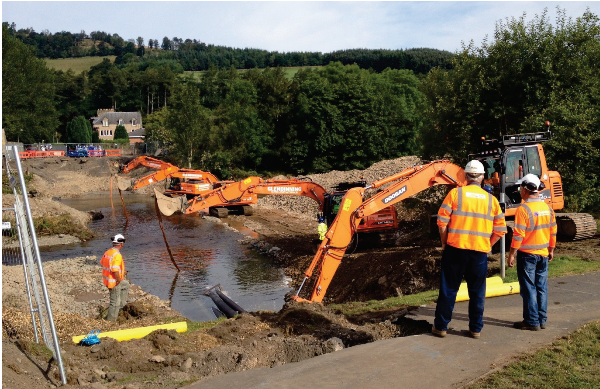
Selkirk FPS – Construction works
