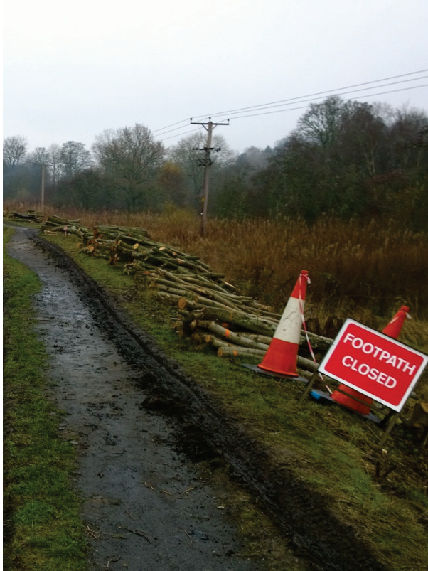
Selkirk FPS – Tree clearance
