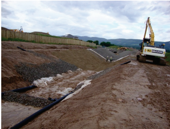
South West Inverness Flood Relief Channel under construction
