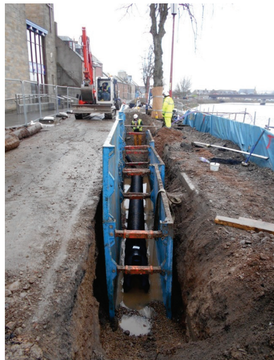
Progress being made on the River Ness Tidal Section
