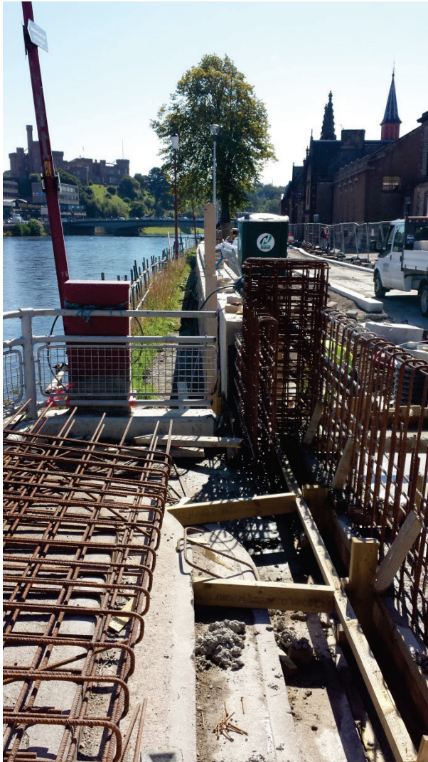
Inverness FPS - Construction work
