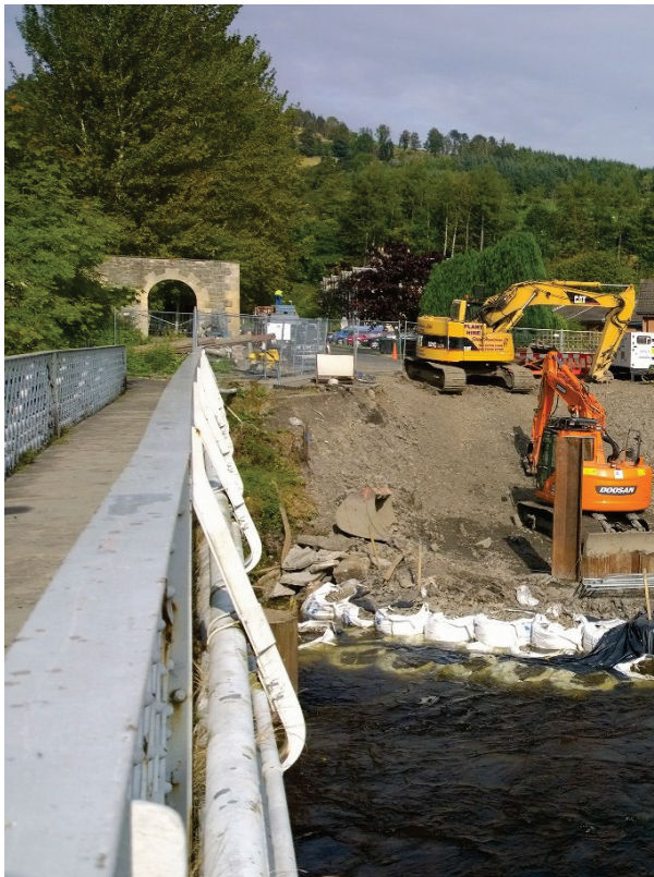
Selkirk FPS – Riverbank construction work
