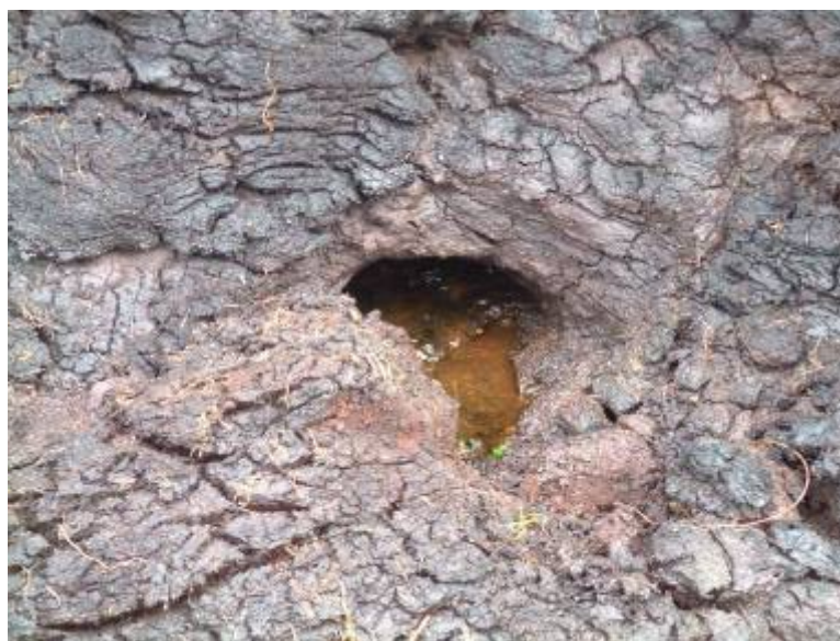
Plate 2.9. Pipe outlet in exposed peat scarp
