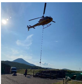
Figure 6: Emergency measures to maintain water supply in Broadford 2023
