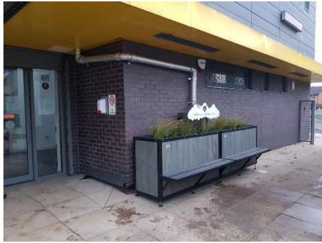
Figure 7: Wellhouse Community Centre, Glasgow – SUDS Planter
