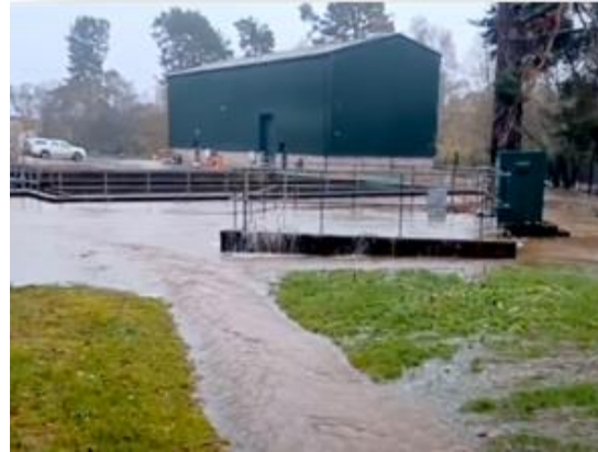
Figure 4: Ballater Water Treatment Works 2022
