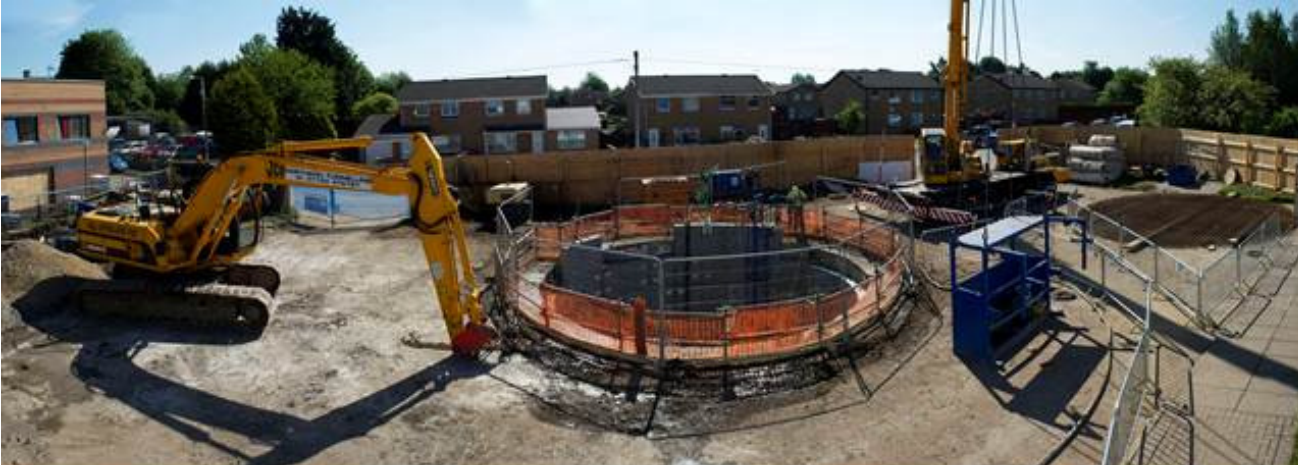
Improvement Underway - Fullerton Avenue Flooding Project, Glasgow
