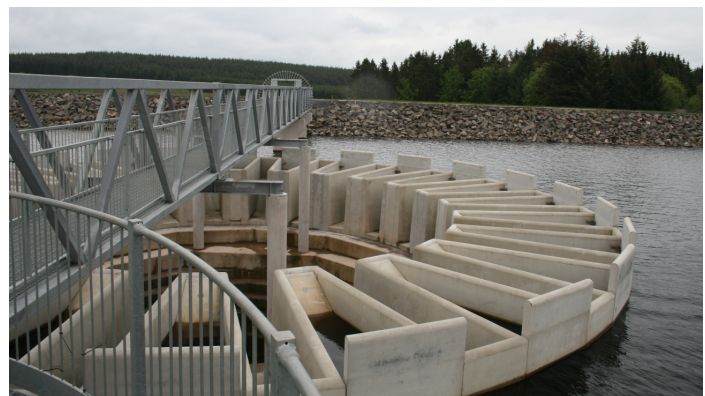
Circular Piano Key Weir Black Esk Reservoir – a world first
