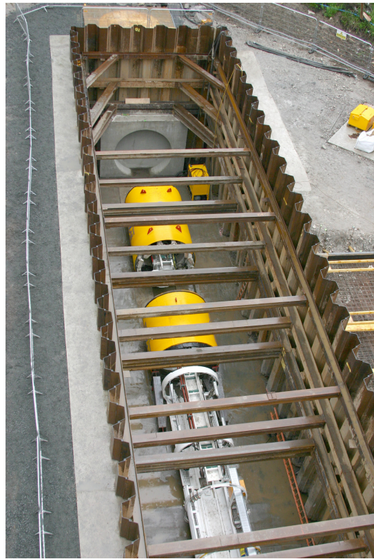
Improvement Underway - Airdrie Tunnel
