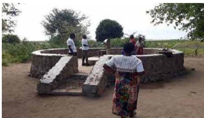
Mapping of a water facility on Chisi Island in Zomba District. Picture taken by United Purpose, implementing partner.
