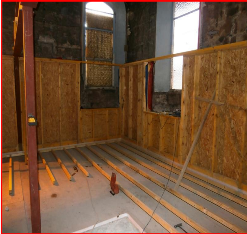
THE CONSTRUCTION OF A 1 ST FLOOR FLAT
