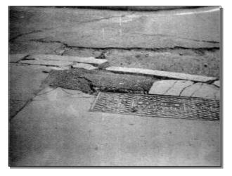
FPCK Failed Patch - adjacent cracking
