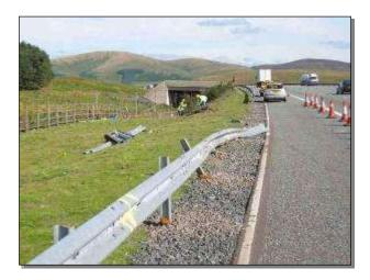
DAMM Damaged Deformed Fence/ Barrier
