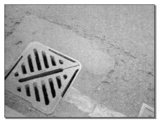
PACK Patch adjacent cracking
