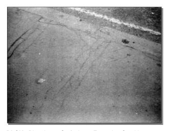
BLCK Bituminous Surfacing – Extensive Cracking
