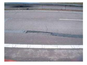
**OVSD** Failed overbanding / sealed cracks
