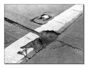
**DSPL** Deep spalling at joints
