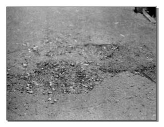
FLMT Failed Patch – loss of material
