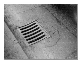
**CKIR** Cracking around ironwork
