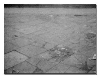
SLCK Slab Cracking
