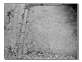
BECK Bituminous Surfacing – Extensive Cracking
