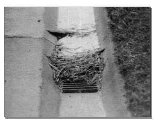
IMWF Impeded water flow
