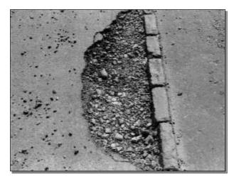
**BPOT** Bituminous surfacing – potholes
