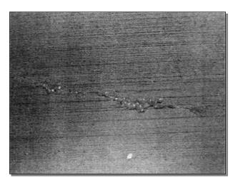
SSPL Shallow spalling at joints/cracks
