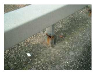
**CMTP** Corroded – metal post (fence / barrier)
