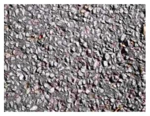
01 Surface: Hot Rolled Asphalt (code 1)
