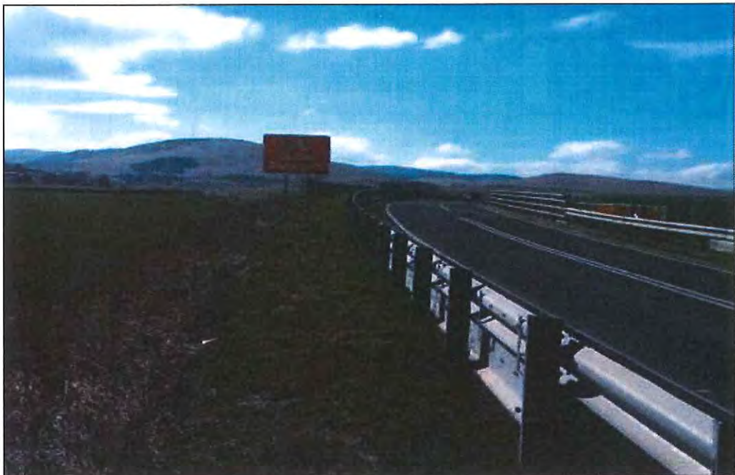
Figure 2.2 – Expansion Joint Warning Signs
