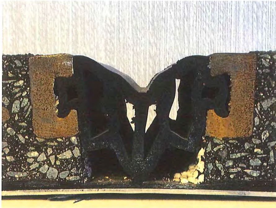
Figure 7: Existing BEJ seal profile
