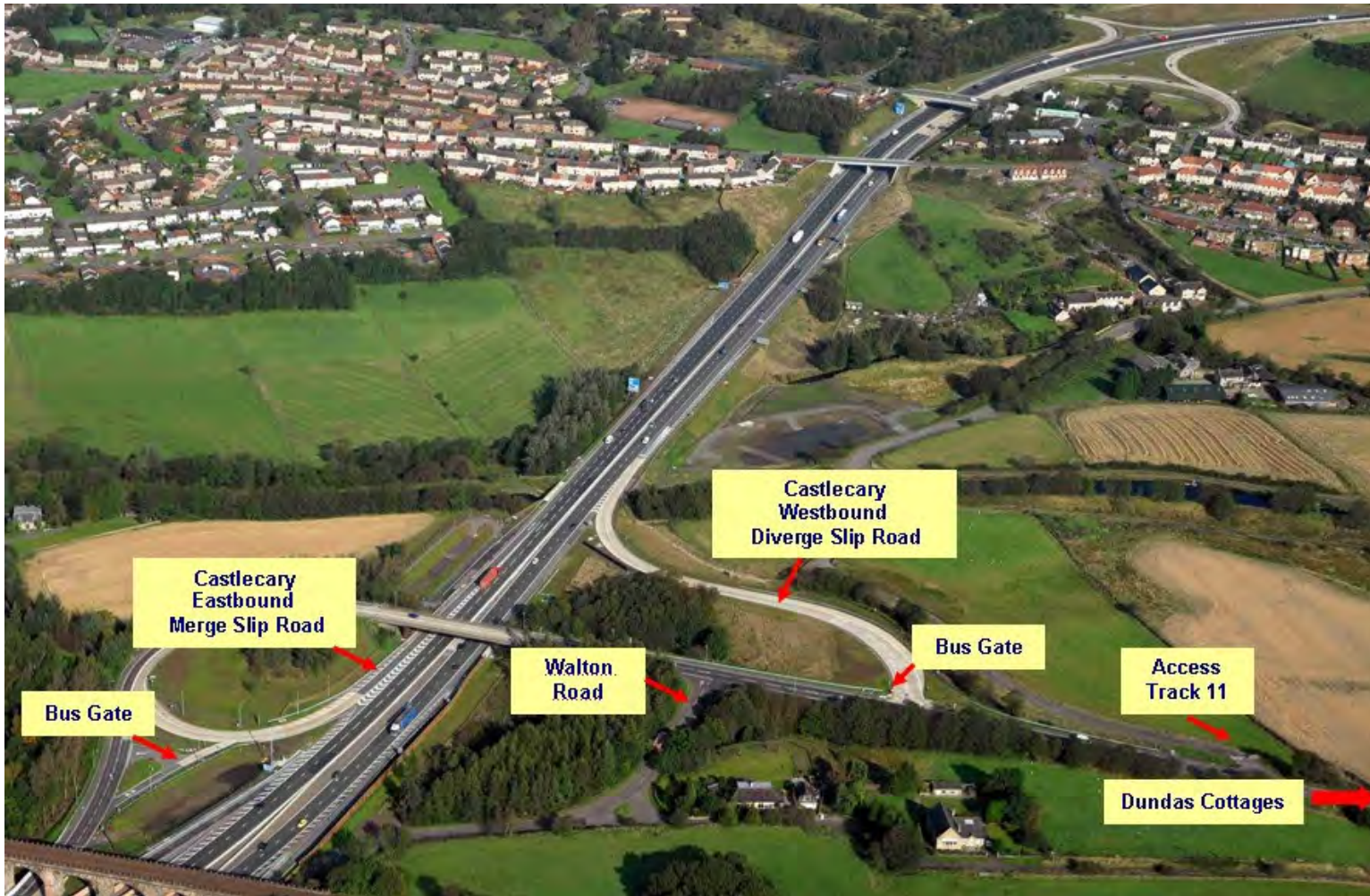
Figure 1: Castlecary Junction – post-construction
