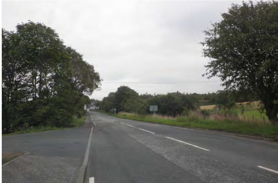
Figure 4: Location of Access Track 11(Post Construction)
