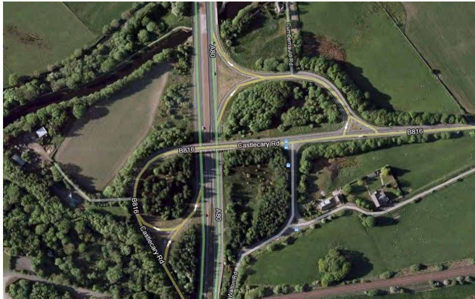
Figure 2: Castlecary Junction prior to Construction
