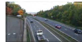
view of bypass from Lanark Road looking across to site
