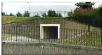
underpass to site
