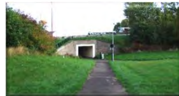
underpass from site
