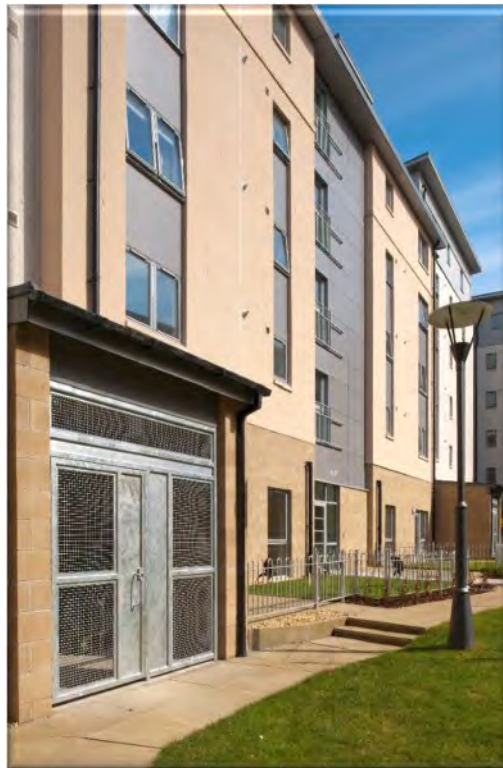
integrated above ground storage areas
