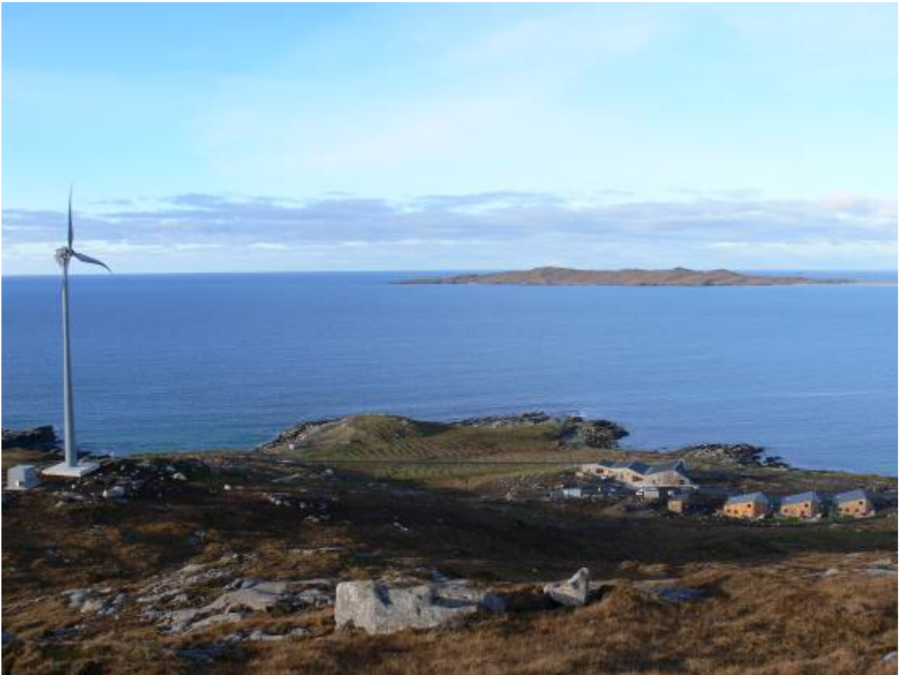
Project nearing completion – photo source: WHT.
