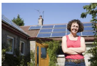
Solar panels (PV)
