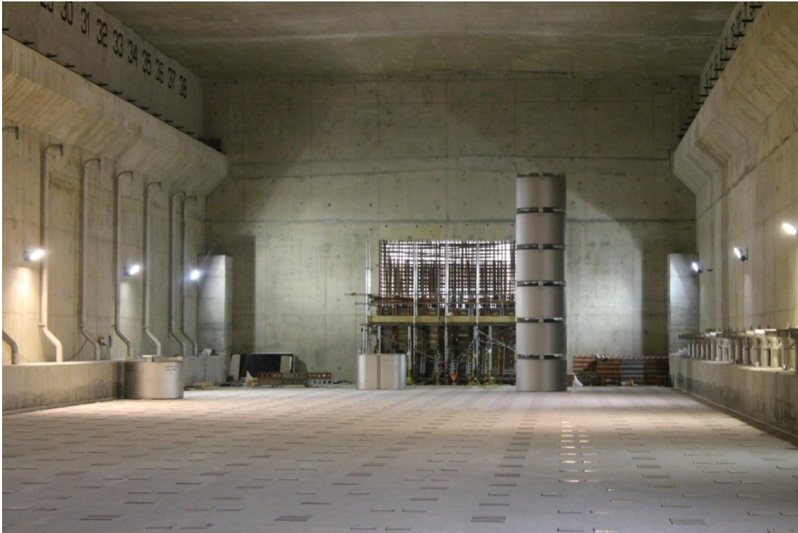
Intermediate Level Waste Storage Facility at Hunterston A
