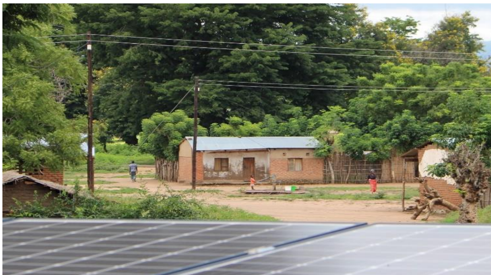
EASE Microgrid Project Photo credit: Aran Eales
