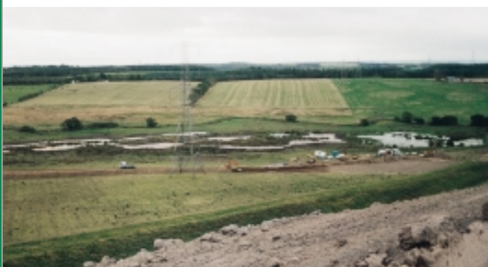
During creation of the wetland area
